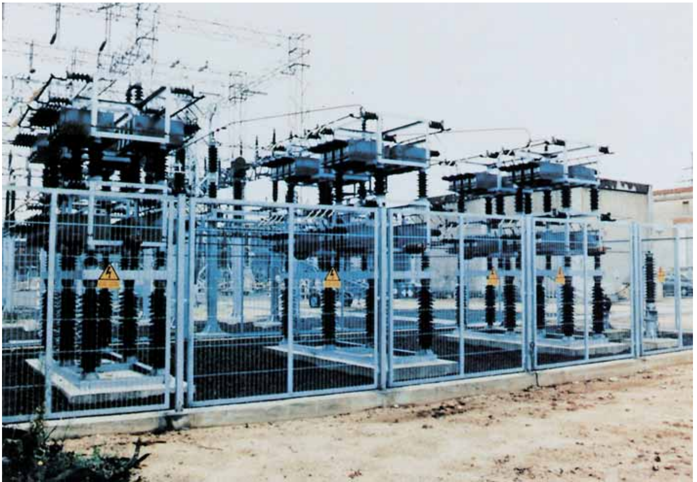
36 MVar - 110 kV - 50 Hz
